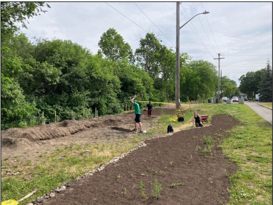
Site preparation. Photo by K. Phillips.
