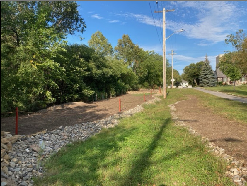
Overview of terraces. Photo by K. Phillips.
